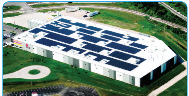
Solar panels powering a manufacturing facility, courtesy of First Solar
